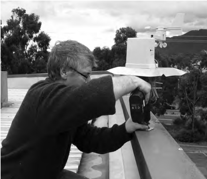
Figure 13-2. Weather station sensors and transmitter being installed
